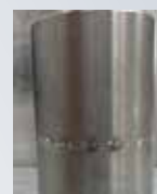
Pipe butt weld Ø 31.75 x 2 mm
